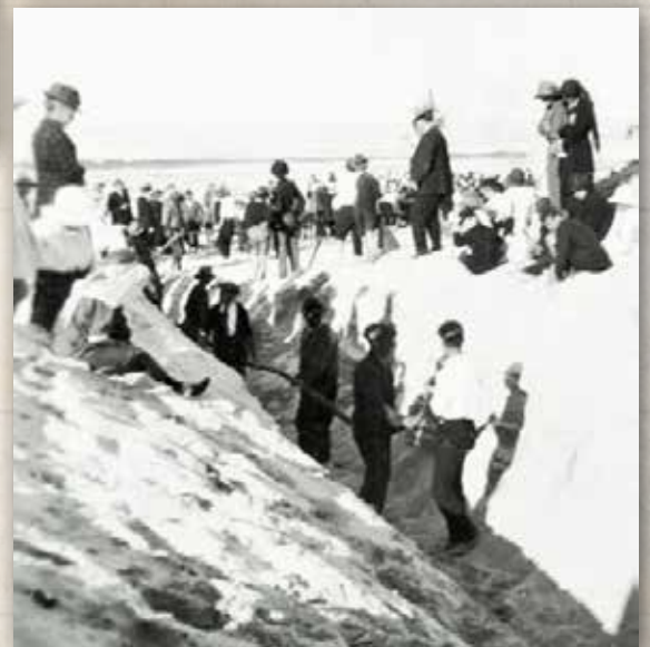
Laying the Pacific Cable in a trench at Main Beach, 1902. Photographer unknown
